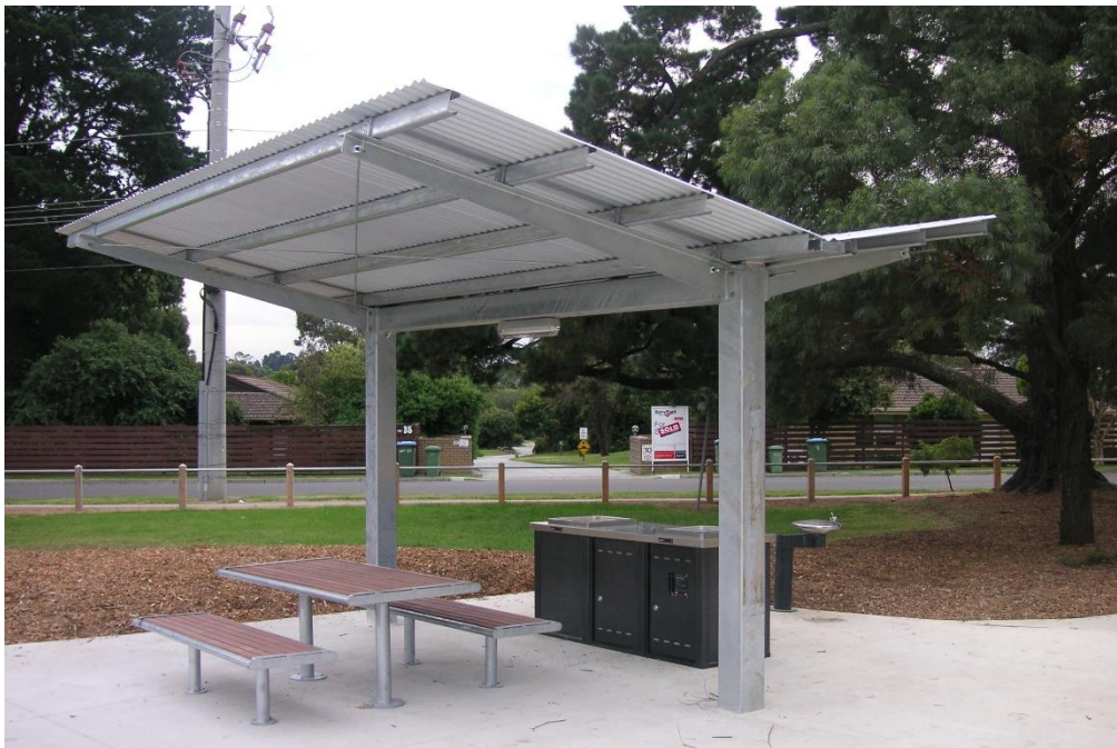
Spencer shelter pictured with hot dipped galvanized supports and Colourbond roof.
