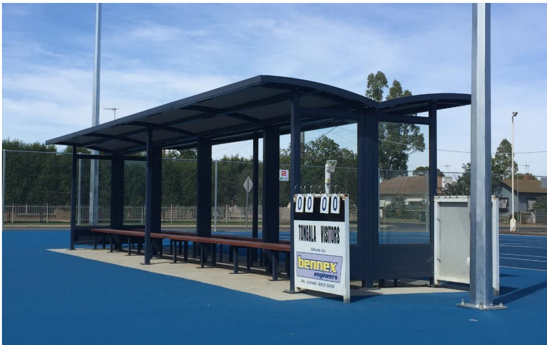
Assumption shelters pictured with safety glass panels and Colourbond roof. Fitted with timber seats.
